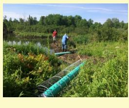
Five years ago, to control the water level from a large beaver dam that resulted in a trail closure, our club purchased a Clemson Leveler (see photo). Developed by Clemson University and field tested by the Minnesota DNR, it changes water flow so that beavers cannot sense it and as a result don't attempt to plug the leveler. Our source in Minnesota for the Clemson Leveler no longer builds them. I decided to create a more robust design, and make them available to ATV clubs.
